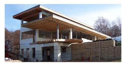
"The thermal mass and airtight construction achieved with the use of Quad-Lock ICF walls and Quad-Deck floors and roof, create a quiet & pleasant atmosphere all year round and that will last for decades to come."
